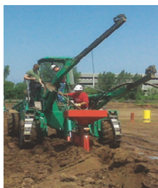
Technology transfer of the Spiderplow to apply to horizontal geoechange allowed 15 km of geoechange piping to be installed in 5 days at a fraction of the cost of a conventional vertical borefield.
