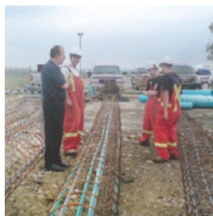
Lead mechanical engineer and piling contractor reviewing how the caisson piles are having geothermal piping attached to the rebar. Photo taken by the lead geothermal engineer.
